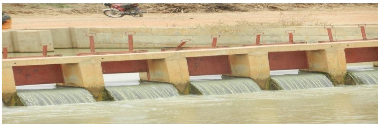
Picture 21: Completed Water Take-off Gate at Hadejia Valley Irrigation Scheme Project
