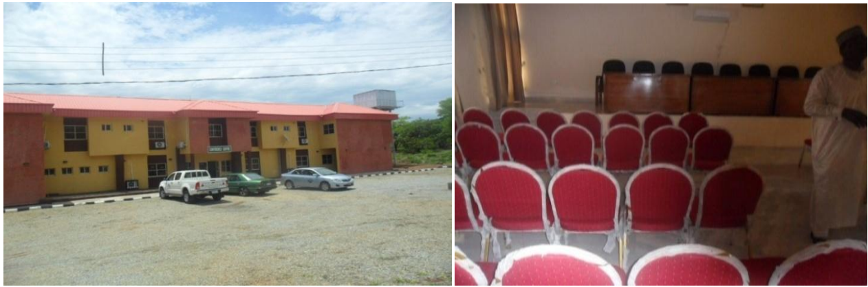
Picture 30: Completed Trainee Students' Hostel, and Part of the Furniture Installed at the Conference Center
