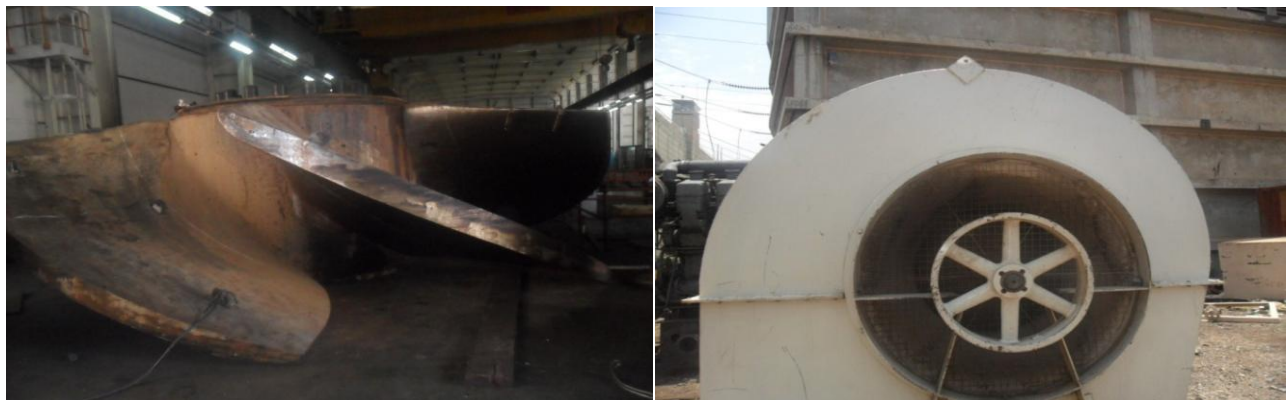
Picture 18: Some of the Dismantled Parts of the Turbines waiting Rehabilitation at the Station
