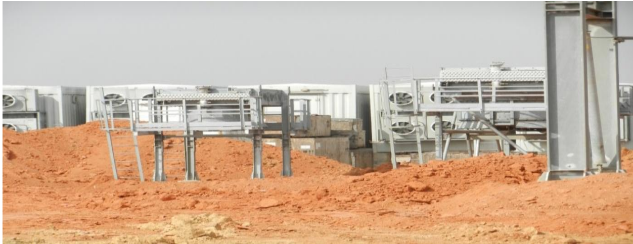
Picture 16: Part of the Delivered Plant Components at 215 MV Dual Fired LPFO/ Gas Power Plant, Kaduna
