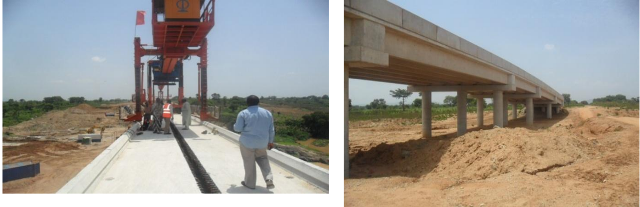
Picture 14: Installation of T-beams at Bridge No.2 (Idu) and a completed Overpass bridges at KM4
