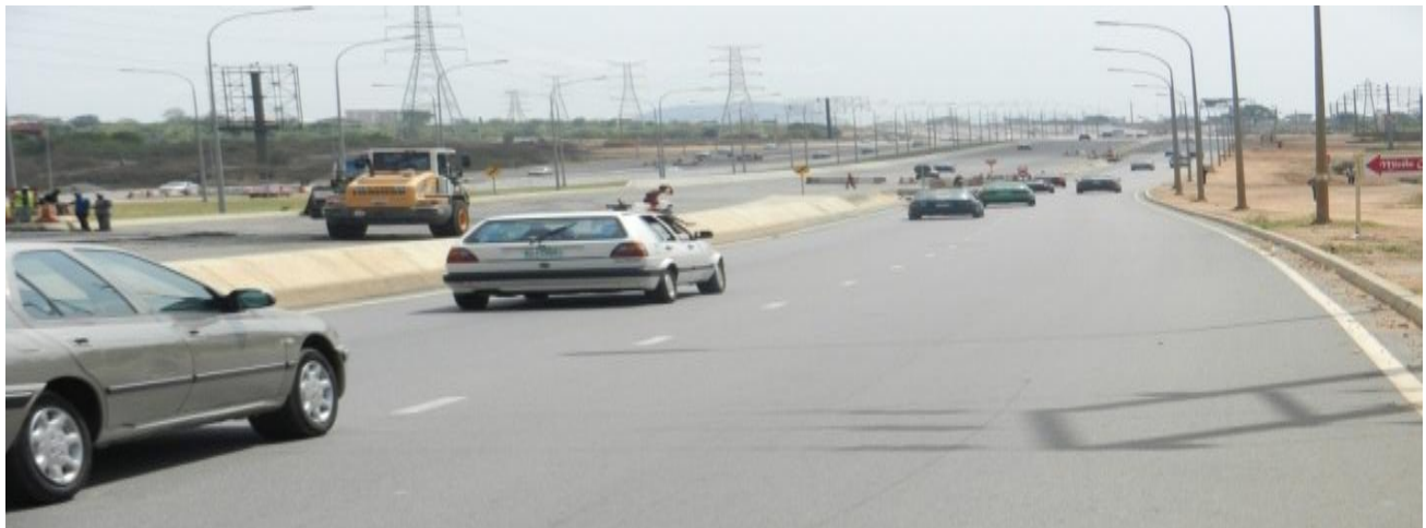
Picture 2: Part of the Completed Portion of the Rehabilitation and Expansion of Airport Express Way Lot 1
