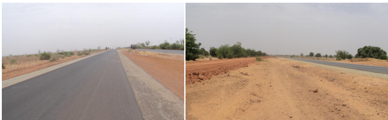
Picture 10: Completed road at section IV and Scarification work on- going at section IV
