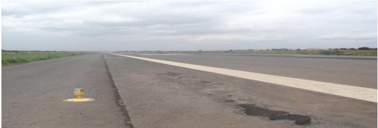
Picture 26: Completed Runway Extension & One Airfield lighting at Enugu Airport
