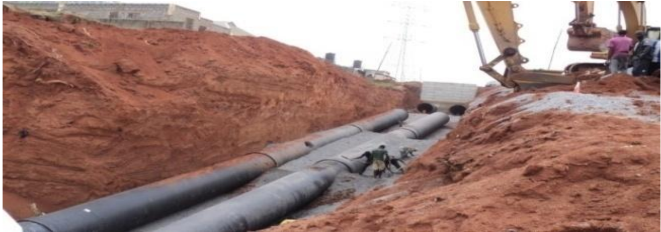
Picture 5: The on-going construction of connecting of Tank 1 & 6 pipes from Lower Usuma Dam Treatment Plant to Tank 1.
