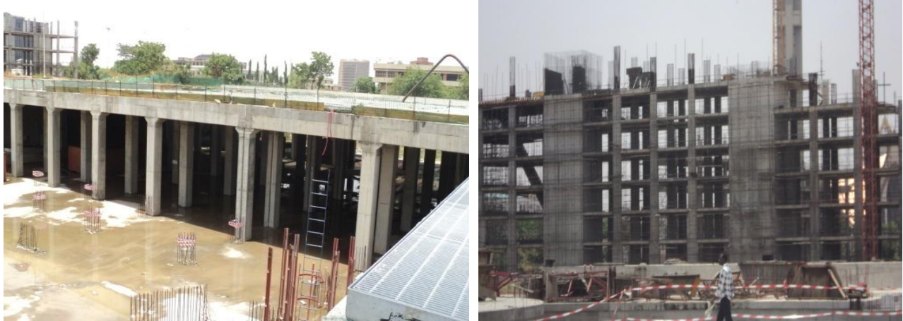
Picture 4: Completed Parking Area and On- going Construction of Hotel
