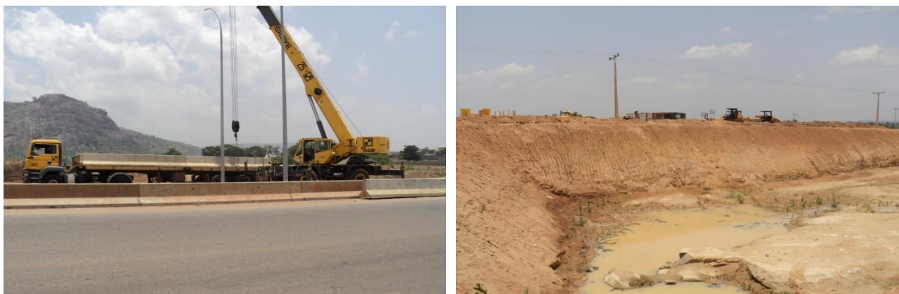
Picture 1: Completed Road and On-going excavation for bridge work at Onex Lot I
