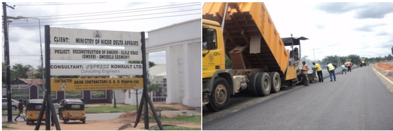
Picture 27: Ongoing Reconstruction of Owerri-Elele Road (Owerri-Omerelu)
