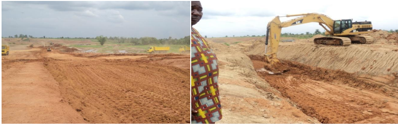
Picture 22: Site Clearance of Dam Axis and Excavation of Key Trench at the New Project Site.
