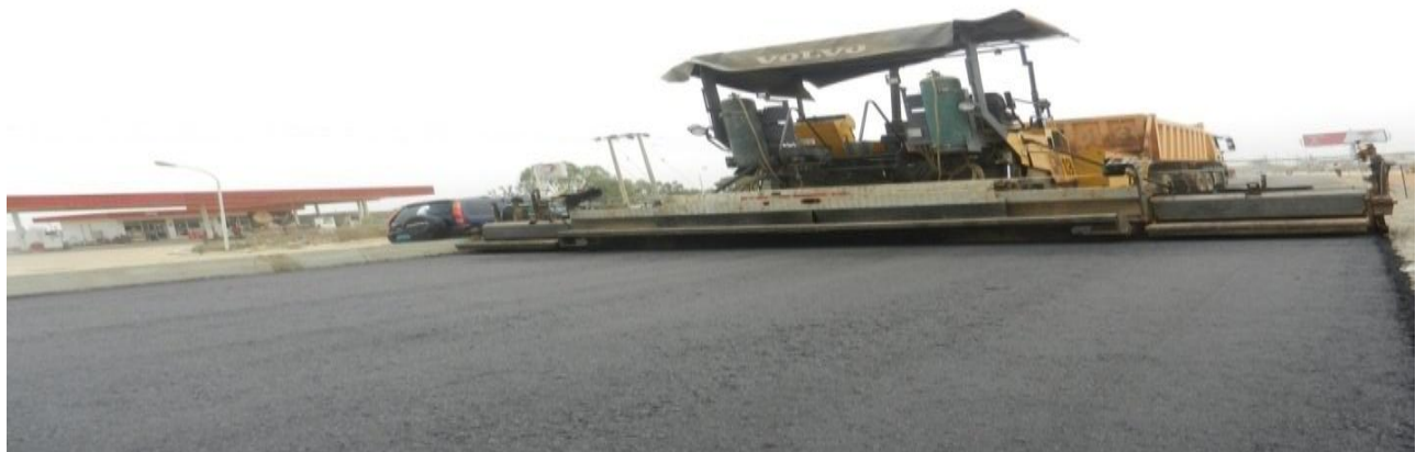
Picture 7: Ongoing construction work at Kano – Maiduguri Road Section I
