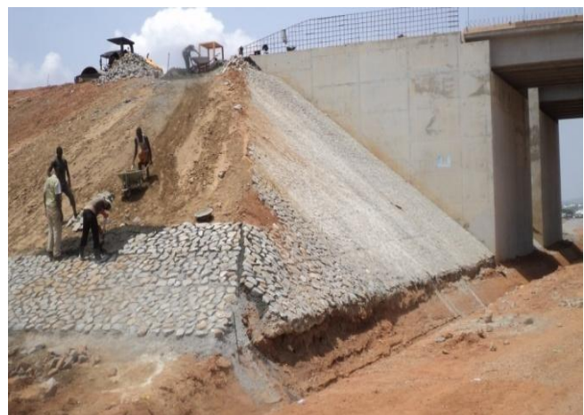
Picture 9: Completed interchange at Giri junction & Stone pitching/Embankment work in progress at the Gwagwalada Interchange
