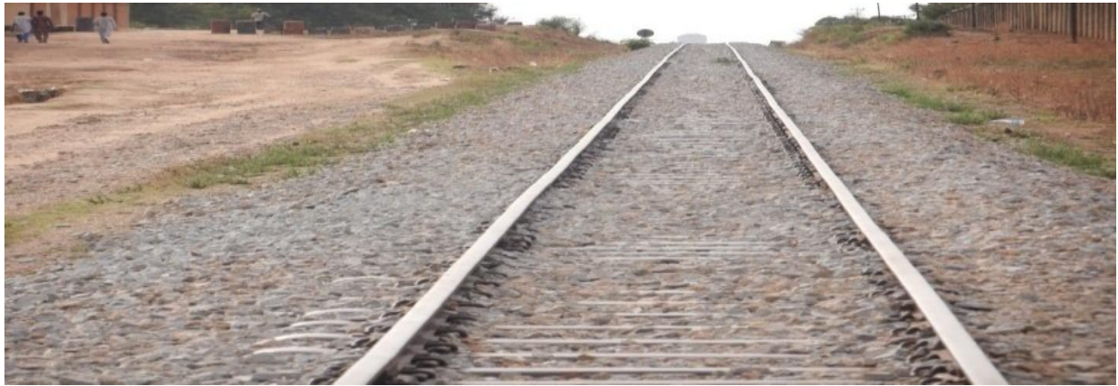
Picture 12: Rehabilitated Track of Zaria – Kaura-Namoda Railway Line
