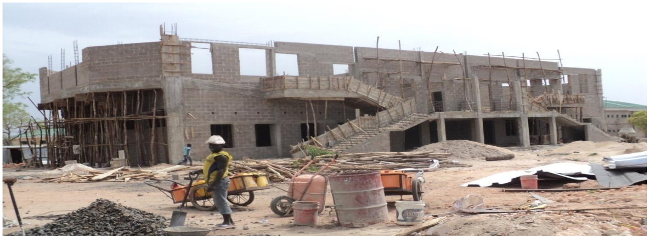
Picture 34: On-going construction of Twin Lecture Theatre and Studios at MAUTY
