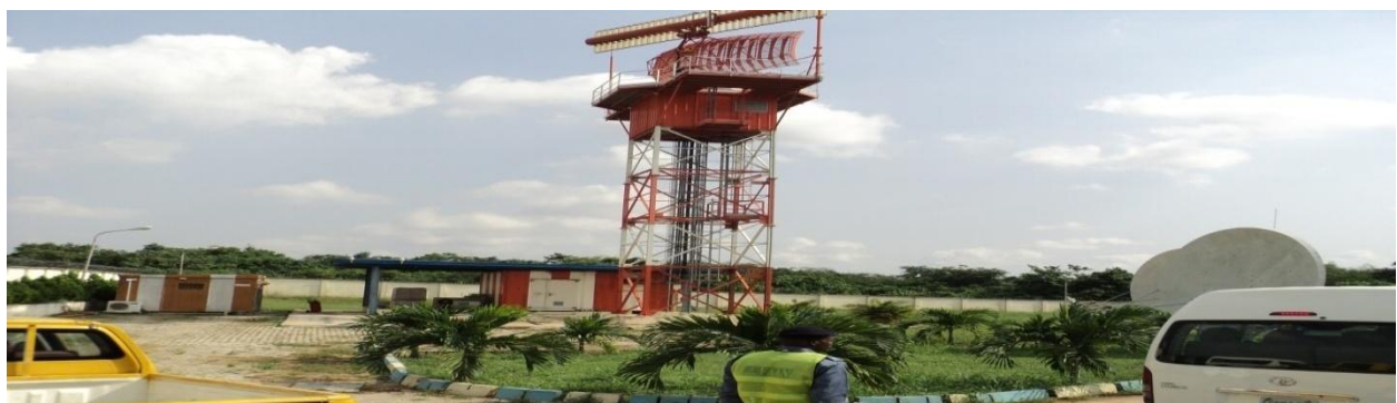
Picture 25: Installed Radar head (Tracon) at NAMA, Headquarters, Lagos.
