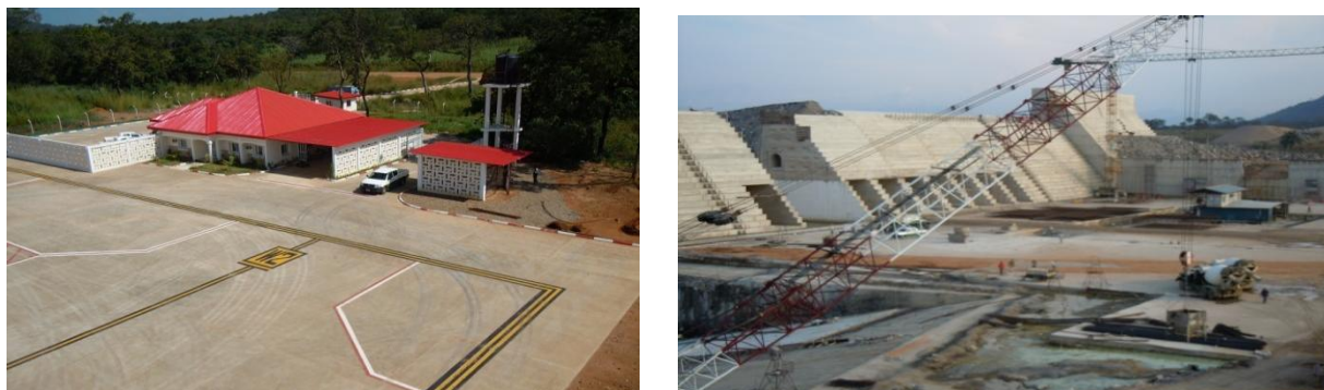
Picture 24: Completed Airstrip Tarmac Building and Spillway works in progress at Kashimbilla Dam
