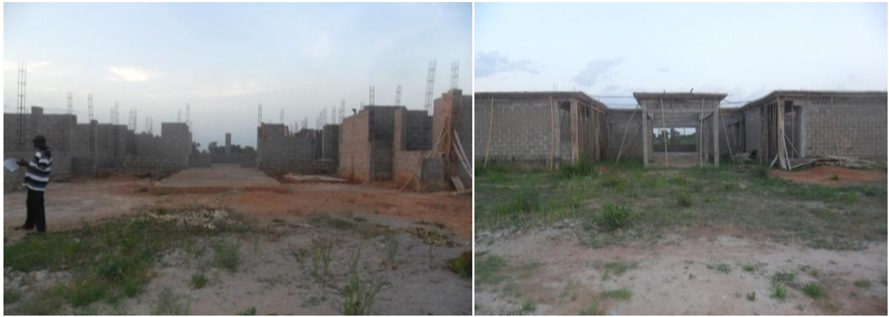
Picture 36: On-going construction of Male & Female wards at FMC Makurdi
