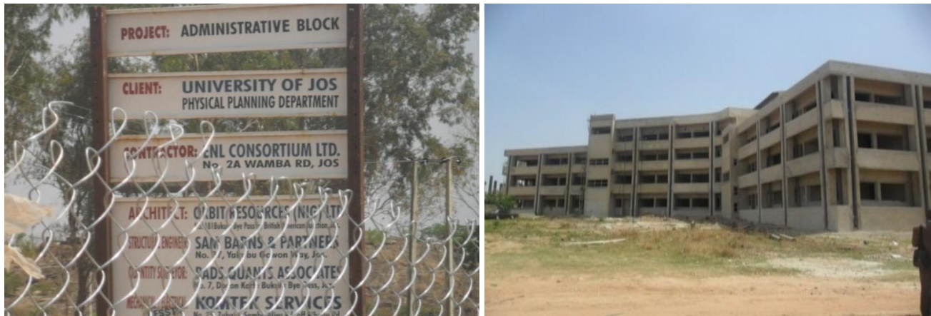
Picture 32: On-going construction of Administrative Block/Senate chamber at the University
