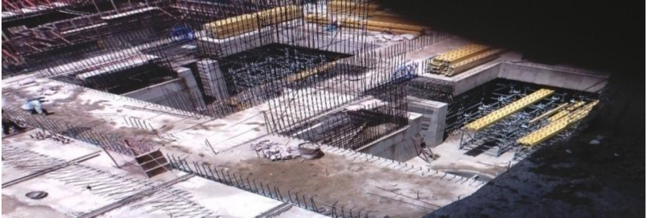
Picture 19: Hydro Power Pit at Kashimbilla Dam
