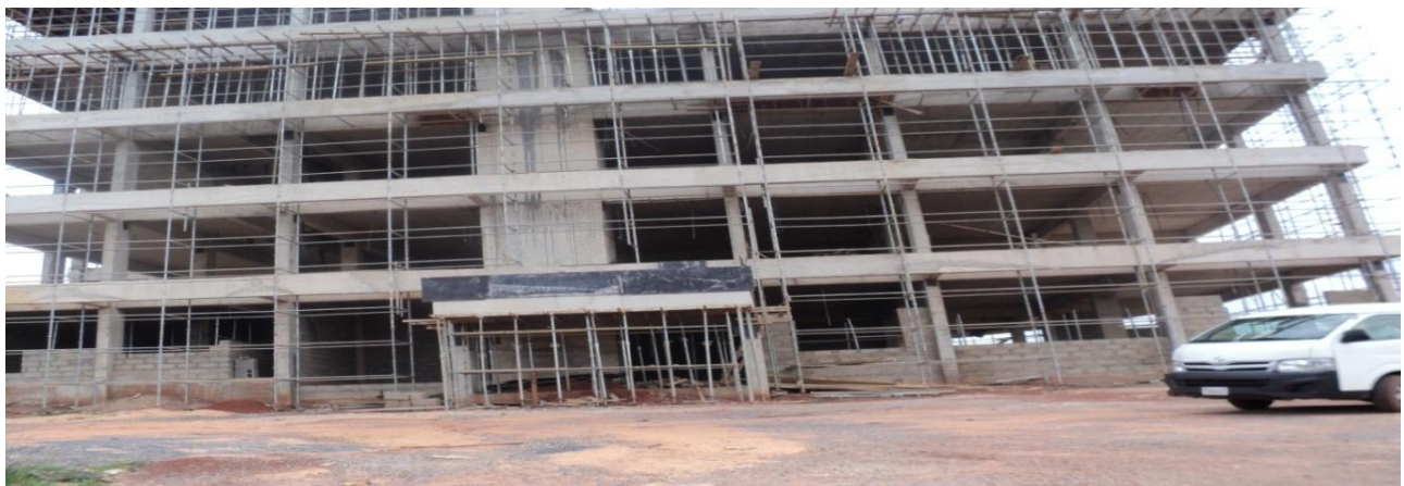
Picture 33: Construction of Administrative Building UNEC Phase1 University of Nigeria Nsukka
