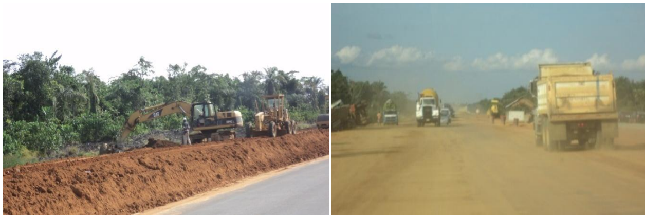
Picture 28: On-going Construction at East-West Road Section II along Port-Harcourt - Ahoada (47KM)
