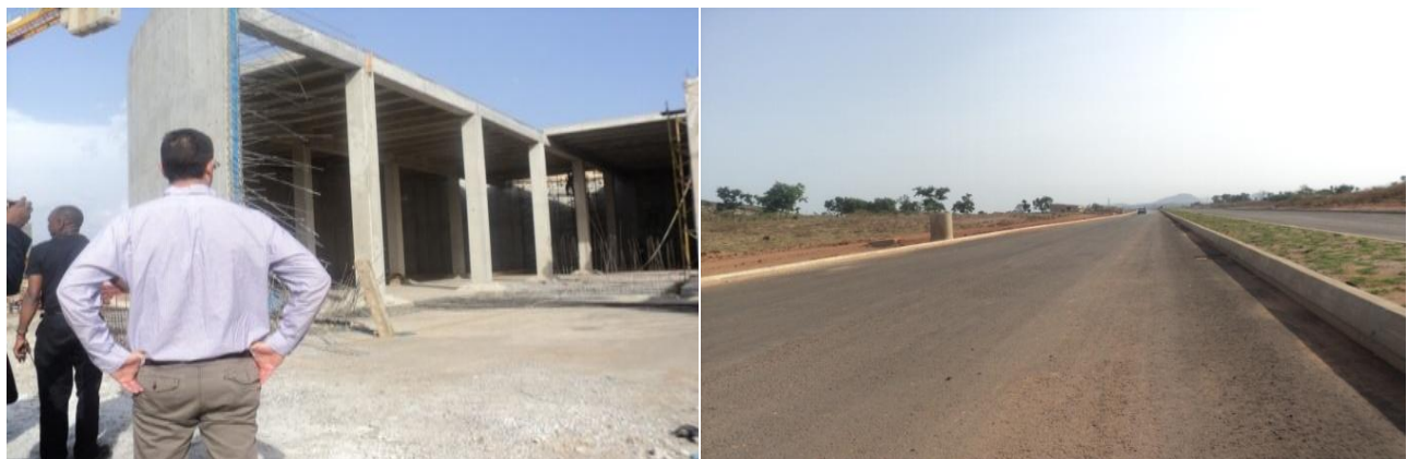
Picture 3: On-going Construction of concrete water tank and Completed access road to the project site
