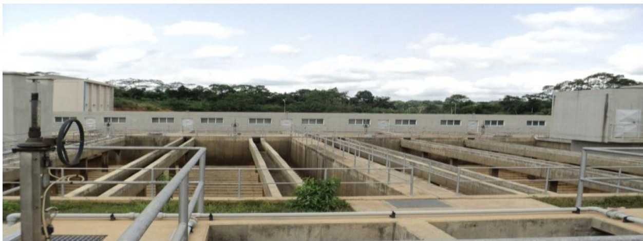
Picture 20: Completed Owena Treatment Plant for Owena Dam, in Ondo State.
