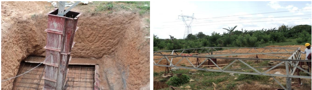
Picture 15: On-going foundation for tower erection at Ede Transmission Line
